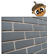
Brickwork finish of GRP
